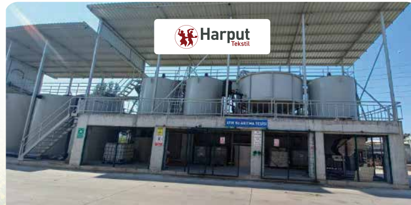
Gökçeköy Weaving Facility /wastewater treatment plant
